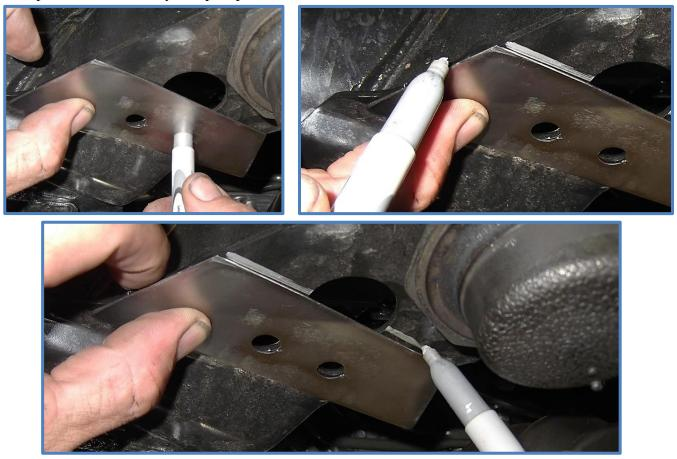
4. Now connect the top and bottom lines on the side of the bracket as shown.
